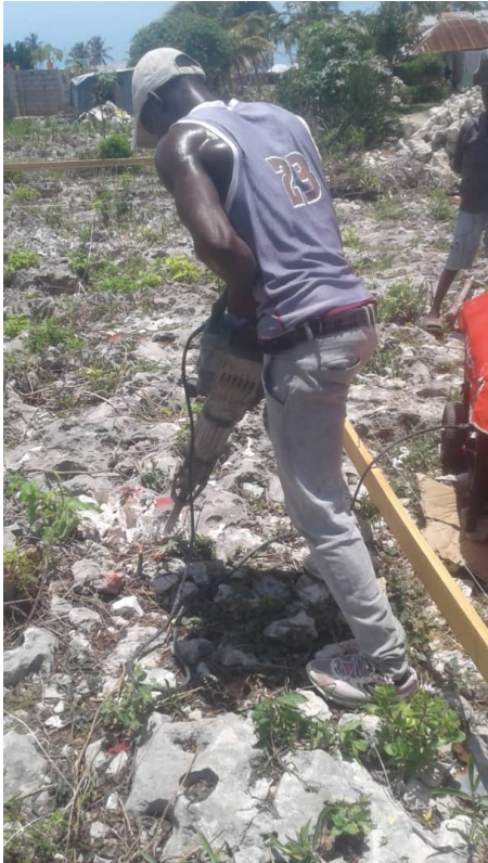
Workers digging rocks to create the foundation for the school construction
