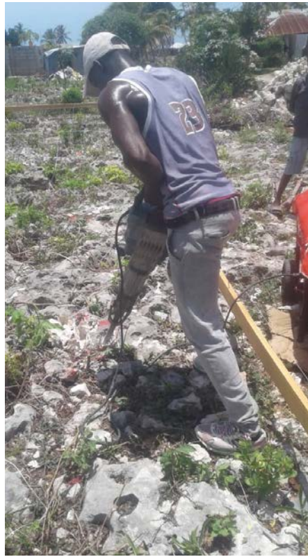
Workers digging rocks to create the foundation for the school construction
